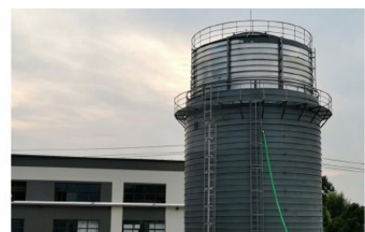
Bell-type gas holder Volume: 500m 3
