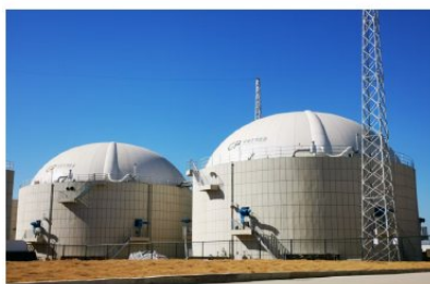
Anhui Green Power Tank-Top Volume:2000m 3 *3,1500m 3 *2
